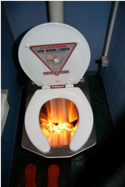
Incinolets Station CONCORDIA
