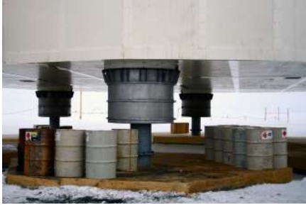
Pilotis hydrauliques Station CONCORDIA
